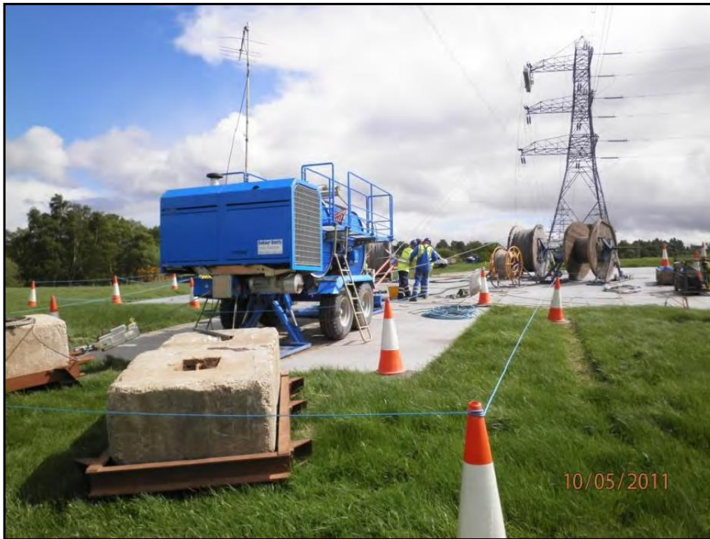
Figure 6.28: Typical Setup for Overhead Line Stringing (Source: SPL)
