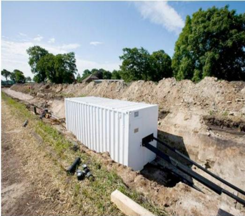
Figure 6.18: Typical Joint Bay Shelter
