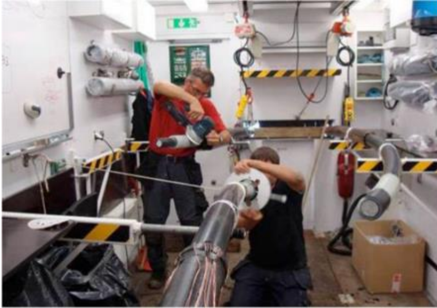
Figure 6.19: Typical Jointing Process
