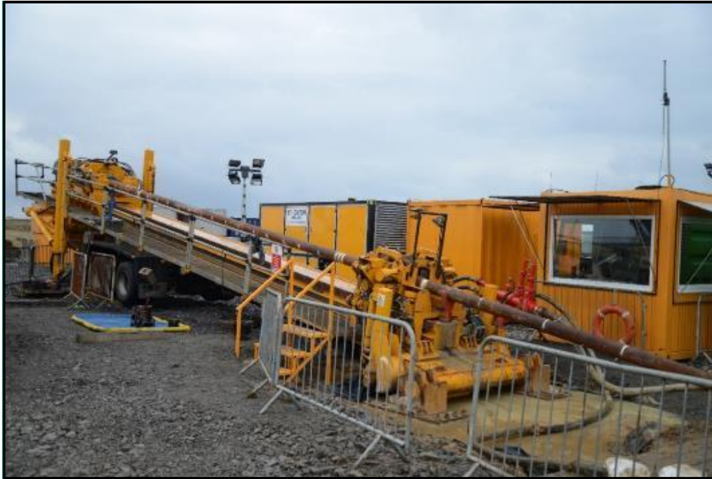
Figure 6.11: Photo of Typical HDD Drill Rig at Landfall
