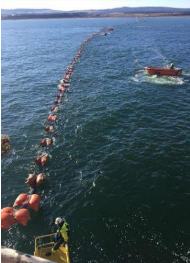
Figure 6.13: Typical cable float in progress
